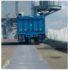
Removing nonskid coatings from a ship deck
